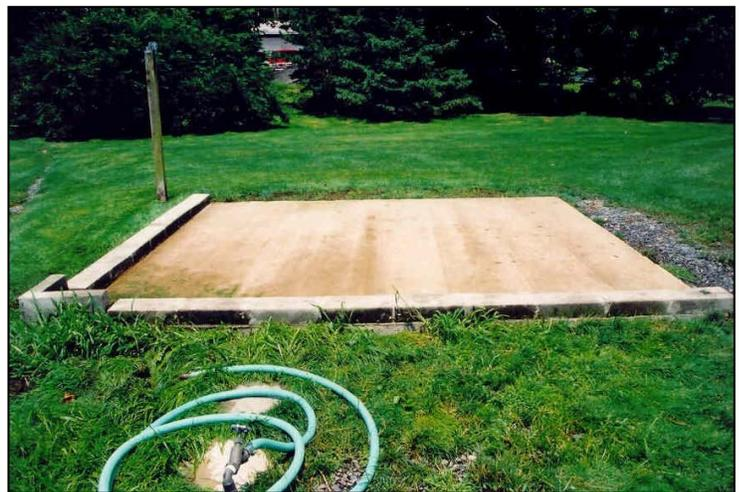
*This wash pad was built for under \$200, which included pouring the concrete, screen, and labor. Cinder blocks were reused from a past project and there is a double screen placed in the lower left corner. Water passes through the screen and out into tall vegetation, which acts as a filter.*
