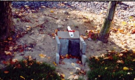
*If a spill were to occur on the chemical mix pad pictured (top), it would drain to the tap pictured (bottom) that can be turned on or off so that spilled product can be captured and reused.*
